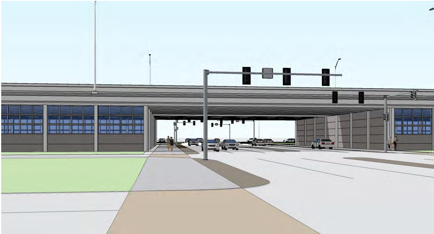
Street View of Elevated I-10 – with Screen Wall and Transparent Tops
