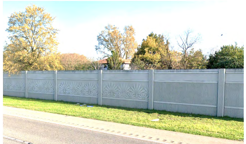
Noise wall with decorative pattern
