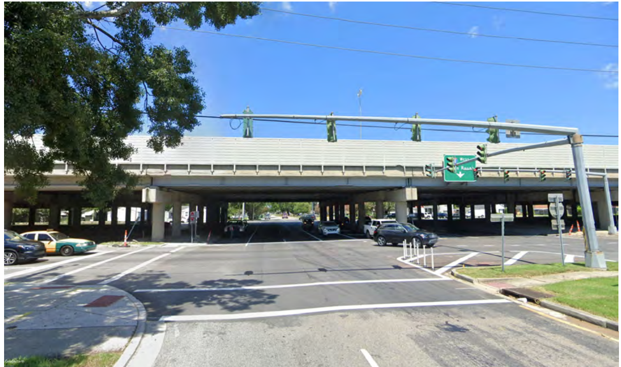
Example of Noise Wall mounted to bridge (I-10 New Orleans)
